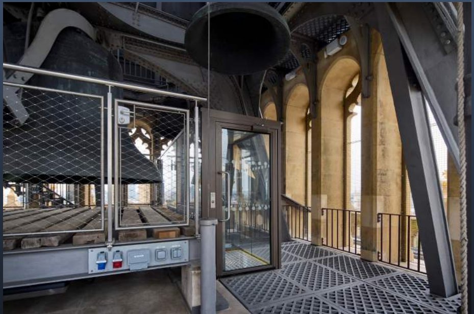
Platform lift nestled within the bells
