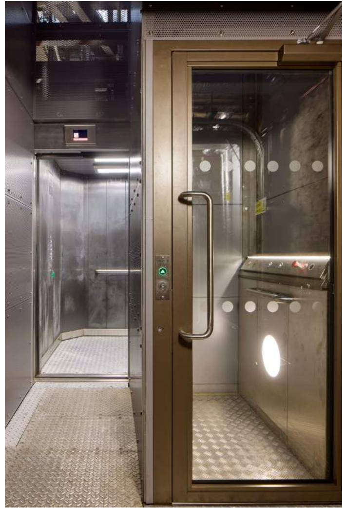
Platform lift access through narrow corridor
