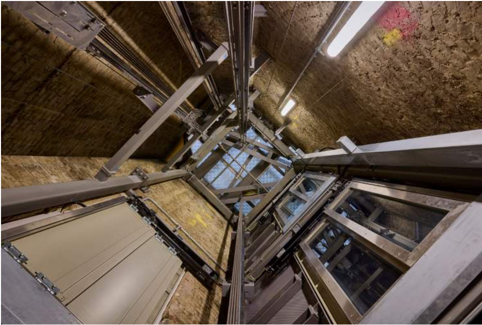
Narrow shaft and structure show the tight tolerances.
