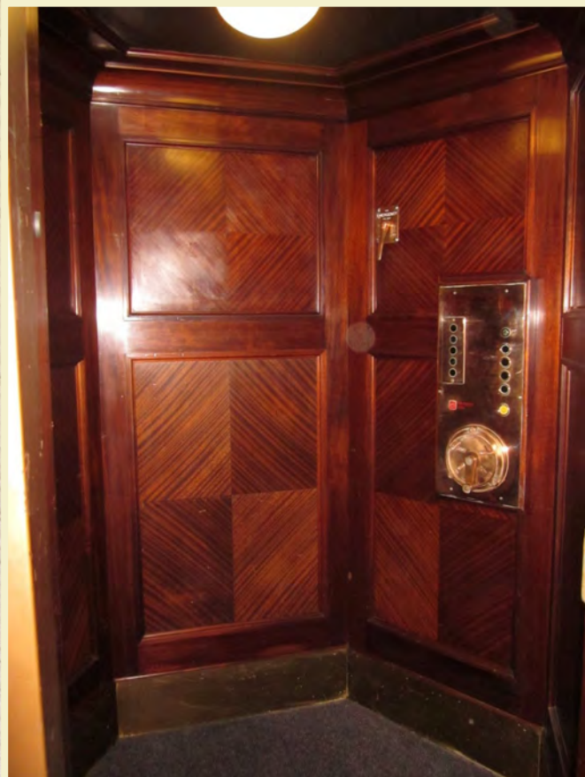
Restored lift car with retained lever emergency stop and attendant control
