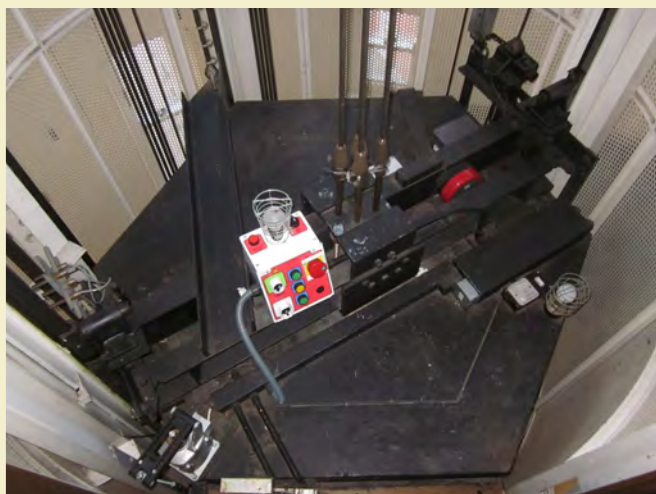
Refurbished lift car for single car entrance and new rope termination
