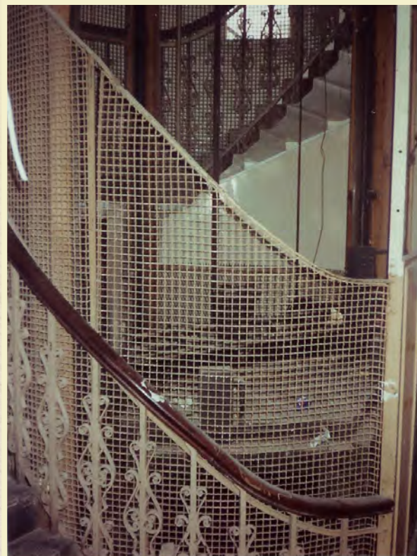
Original shaft enclosure
