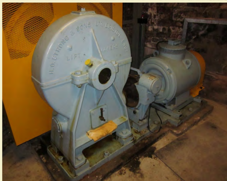
Restored lift machine still in good condition 30-plus years after restoration
