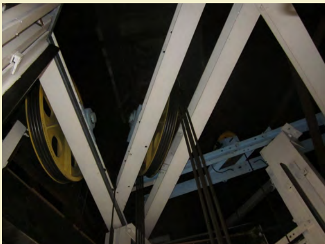
Restored overhead pulleys and new car overspeed governor
